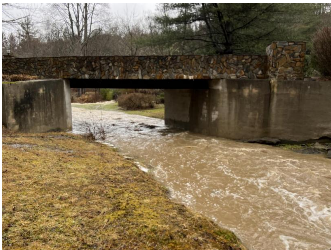
Rocky Creek Bridge
