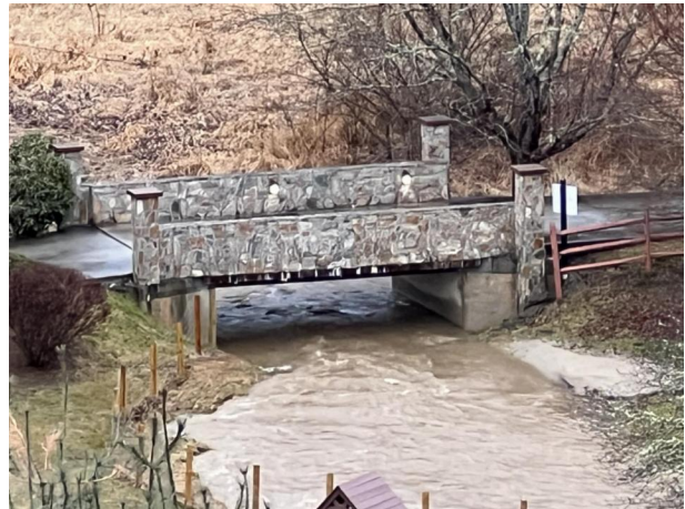
Old Barn Rd. Bridge
